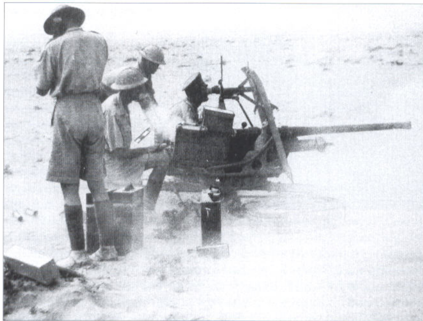
The British 2-pdr Mk I AT gun weighed 1,858lb, about twice as much as its US and German 37mm counterparts. It could be fired from its wheels, but they were normally removed for action and the gun set up on its integral three-legged mounting. Side shields were available, but seldom used.
